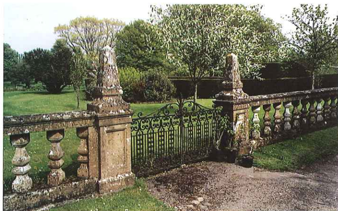
BALUSTRADES, PERROTT HILL SCHOOL
